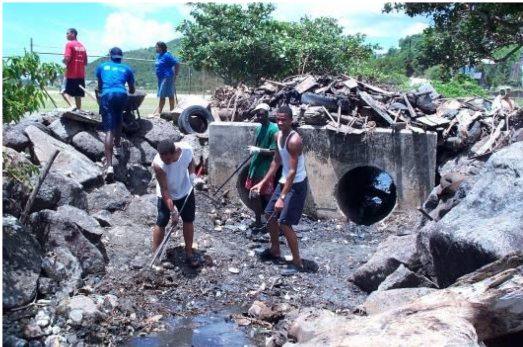
The culverts became visible after several hours of work, and tons of garbage removed
