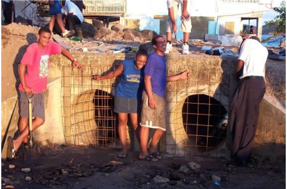
Constructing debris traps
