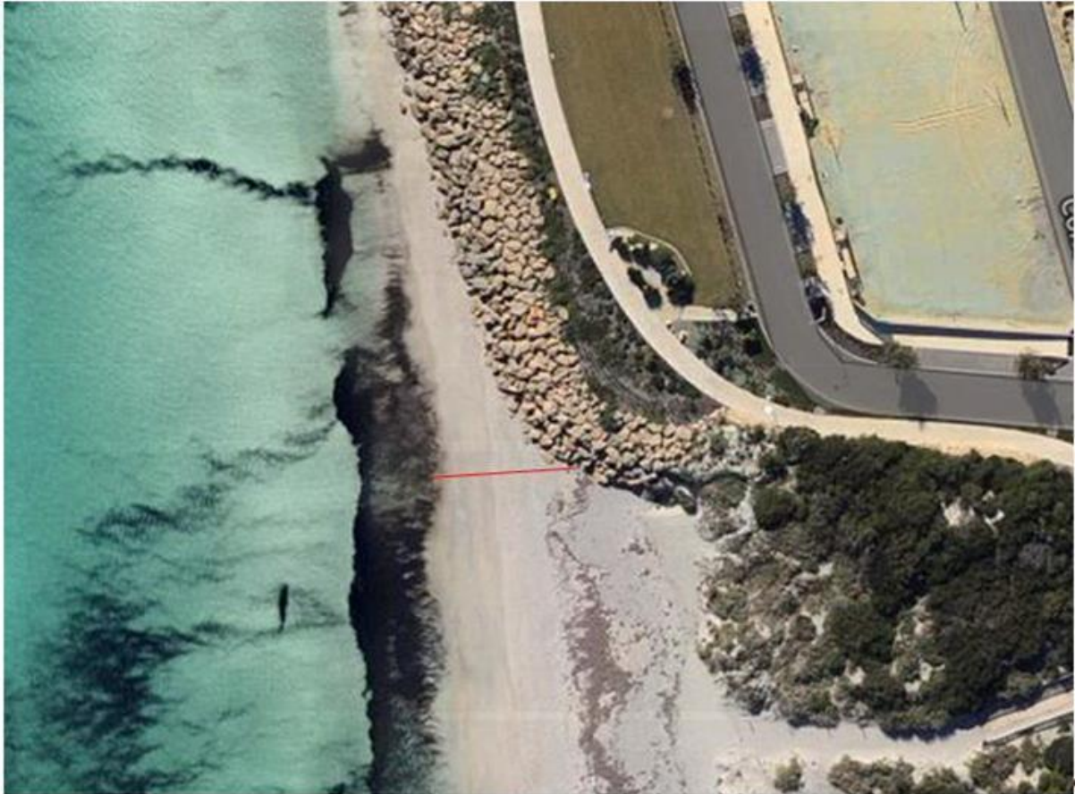
Site 3: Port Coogee Sea Wall
