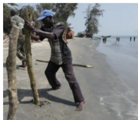
Figure 5: Stake driving technique
