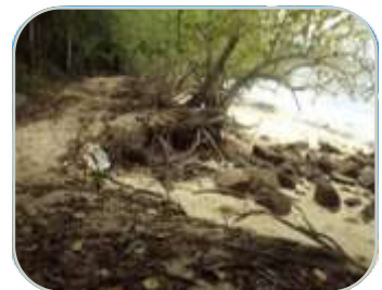
The erosion of the old coastal road is all too plain to see.
