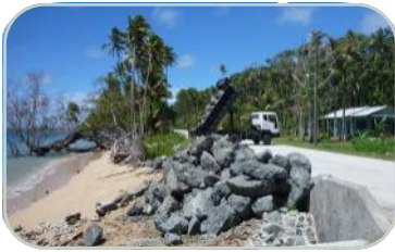
Boulders being placed along the road in Babeldoab after the passage of Typhoon Bopha
